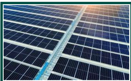
Commercial/Industrial Rooftop Solutions
